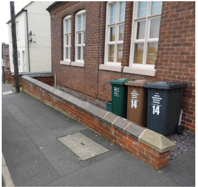
Above left - salt-glazed, bull-nosed copings to dwellings at Church Street are a rare survival and salt-glazed saddleback copings have been restored (above right) at 12-16 Coppice Side under the recent partnership scheme. At present, sections of these walls could be removed without planning permission.
