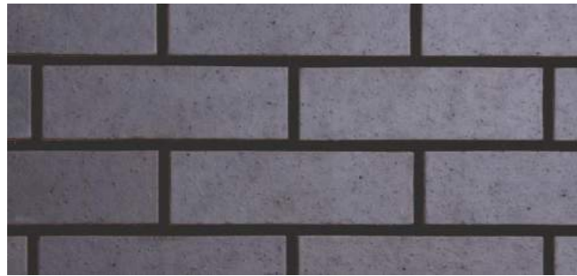
Staffordshire blue clay bricks making up curved planters
