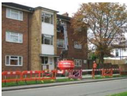
Gutter clearing by local builders, Harvey & Clarke
