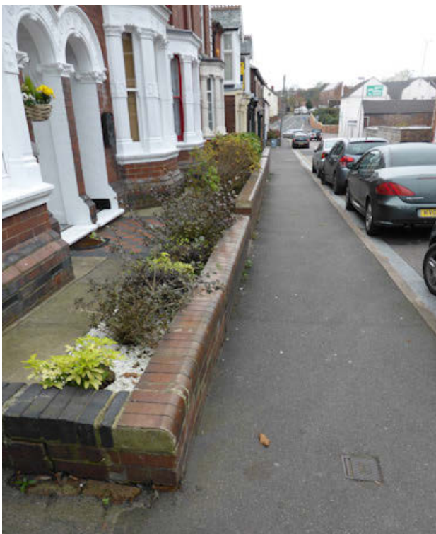
Above left - salt-glazed, bull-nosed copings to dwellings at Church Street are a rare survival and salt-glazed saddleback copings have been restored (above right) at 12-16 Coppice Side under the recent partnership scheme. At present, sections of these walls could be removed without planning permission.
