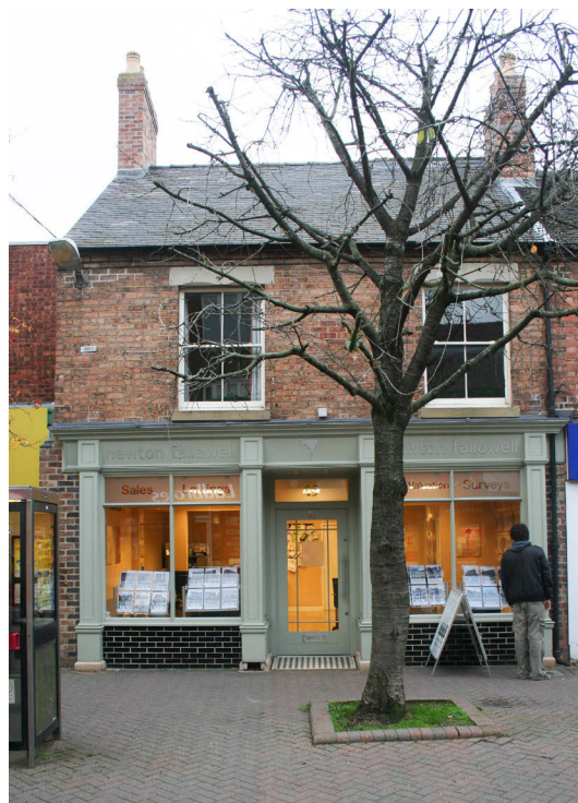
2005 - left and 2014 - right. A willingness on the part of the shopowner at 71 High Street has transformed the shopfront and improved its street presence. The main shopfront has been restored with a new mullion and recessed doorway with a hand-painted fascia, but it is the change to the colour scheme and internal lighting which has had the greatest impact.
