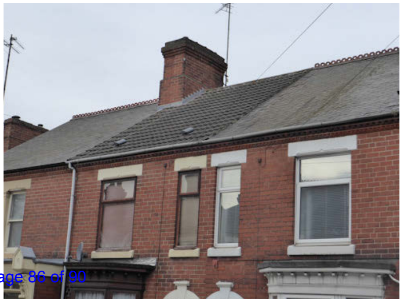
Right - the replacement of Welsh slate roofs with concrete tiles is a major loss to historic character. This example on Church Street stands out in a uniform roofscape. Alterations like this, to domestic properties, are currently permitted development.
